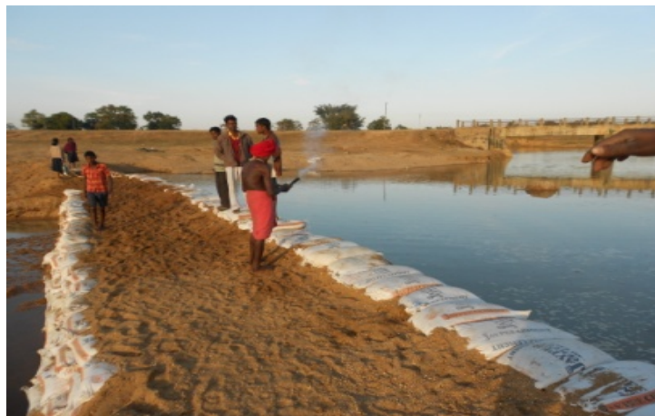
Construction of Sand Bags Check Dam by Villagers
