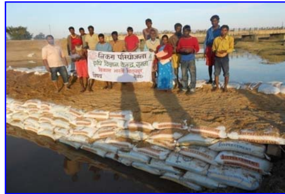
Sand bag check dam built by shramdaan
