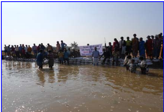
Sand bag check dam built by shramdaan
