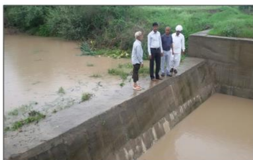
Rain Water Harvesting Structure
