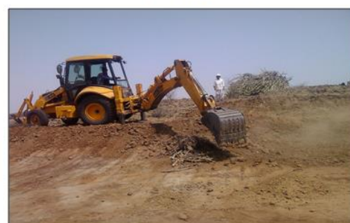
Desilting of Checkdam
